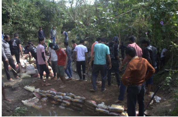
Construction of "Vanrai Bandhara"
